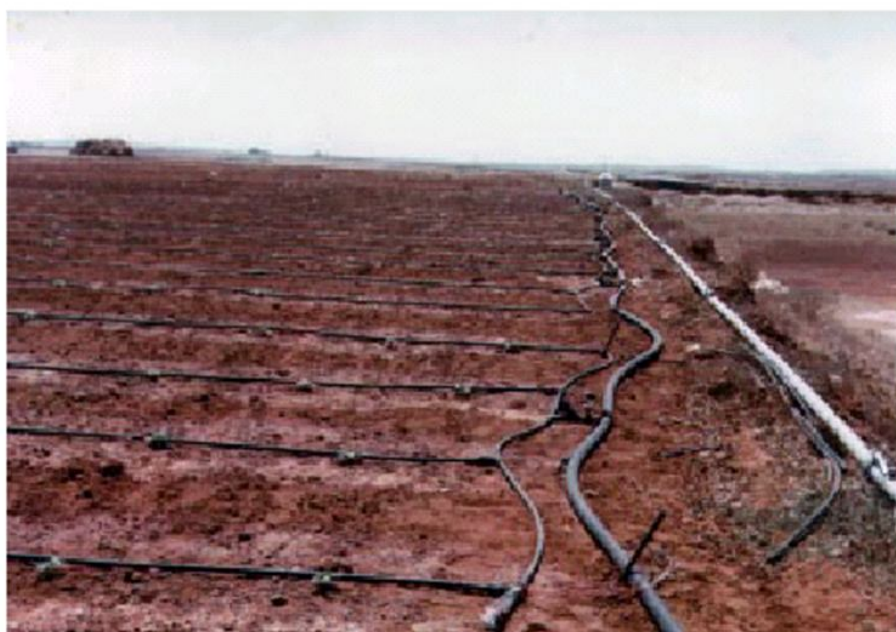
The mains, manifold and dripper laterals
